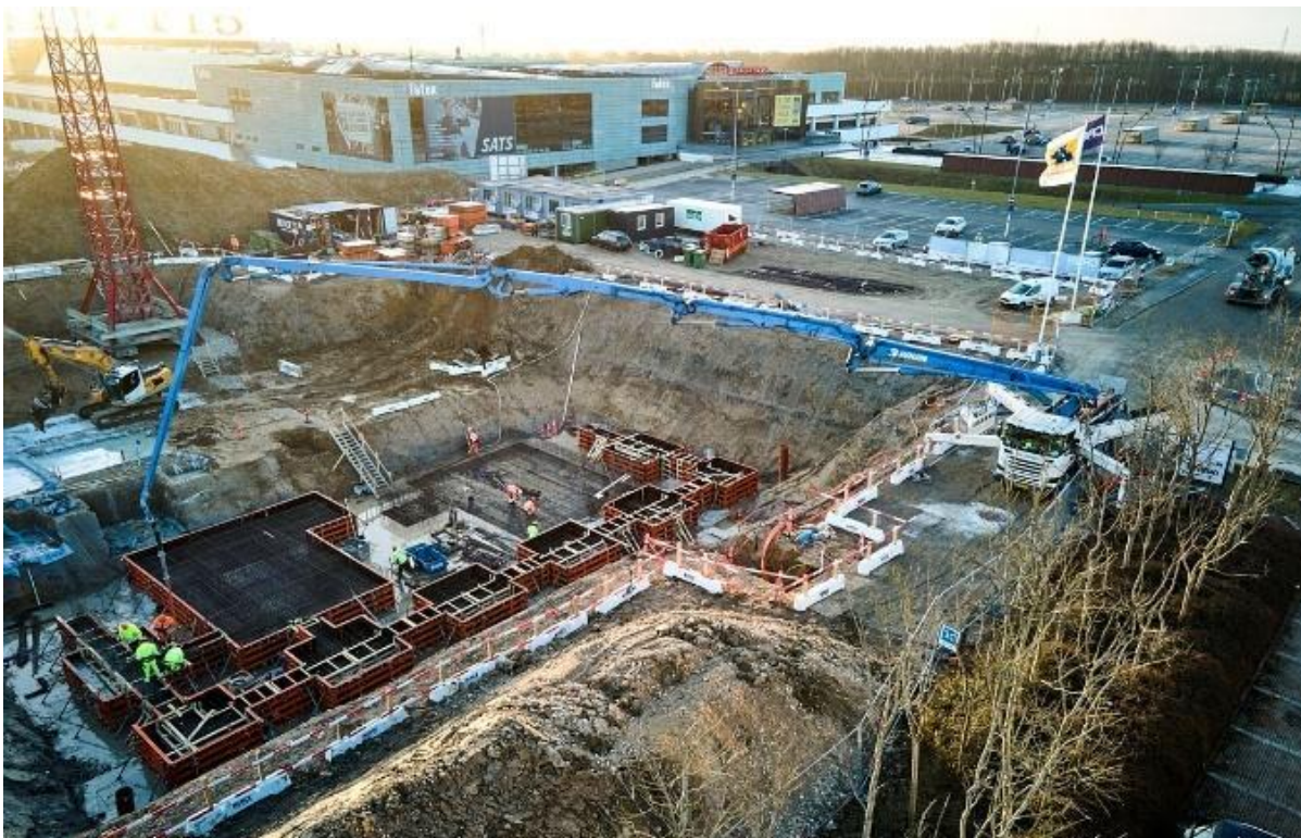
Pouring of concrete foundation with 100 % recycled aggregate, photos: Unicon
