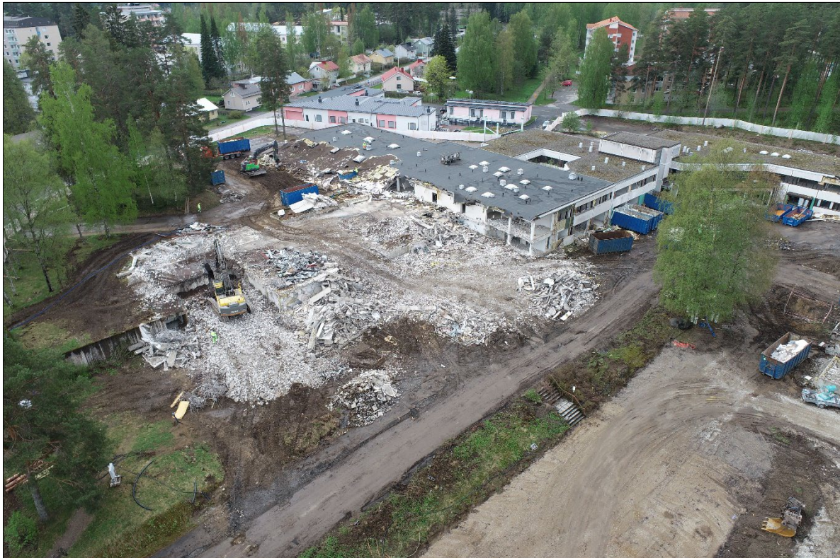
Figure 1. Pankalampi Health Centre during demolition. (Picture: Juha Vihavainen)
