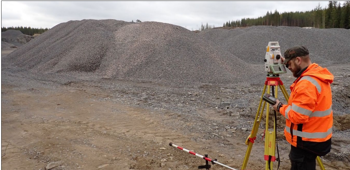
Figure 9. Volume measurements from a material pile. Tuomas Kellman from Maanrakennus Talpa Oy is making volume measurements with a tachymeter. (Picture: Juha Vihavainen)
