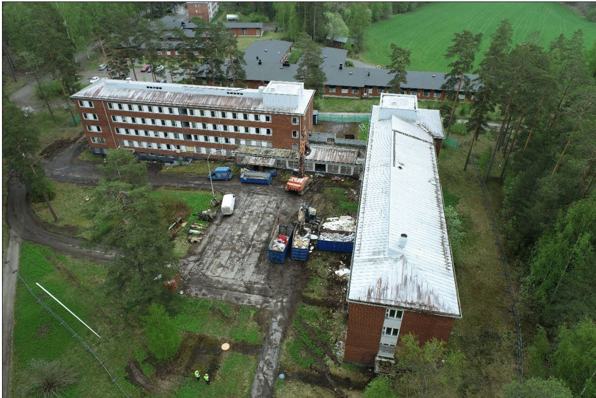
Figure 2. Tuukkala Hospital during demolition. (Picture: Juha Vihavainen)
