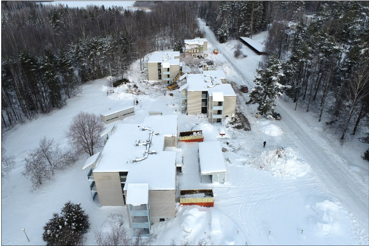
Figure 3. Pellosniemi residential buildings during demolition. (Picture: Juha Vihavainen)
