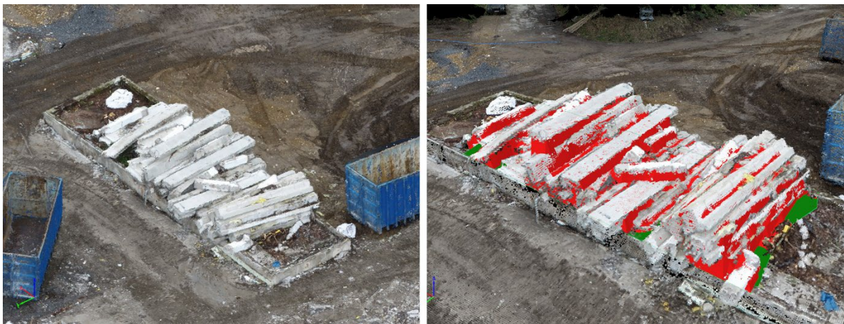
Figure 19. Volume calculations from a pile of concrete beams.
