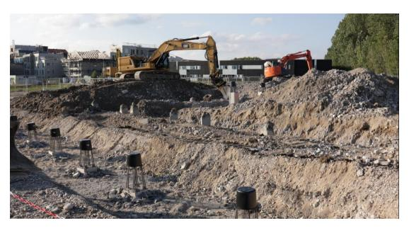
A criterion in the tender for the new car park was that the developer implemented design for disassembly, including scenarios for future recycling. Consequently, a report was delivered by the contractor (MT Højgaard). They created the multi-storey car park with a steel skeleton, premade components assembled by bolts and a minimal use of concrete.
