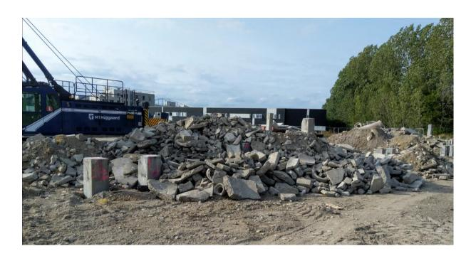
In this case, instead of the above-described normal procedure, the contractor was to contact the builder, agree on excavation, and place the excavated concrete waste just outside the plot. The contractor would then continue with his normal tasks, while the project manager of the builder ordered a crushing contractor to crush and sort the dug-out materials into three fractions. Fine, coarse and mixed aggregates.
